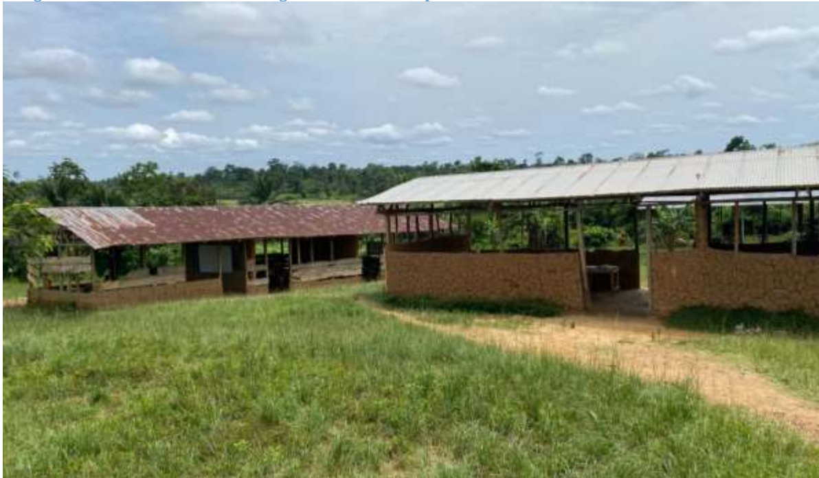
Figure 4 - The condition of Assin Ningo D/A Basic School prior to the construction of the 6-unit classroom block
