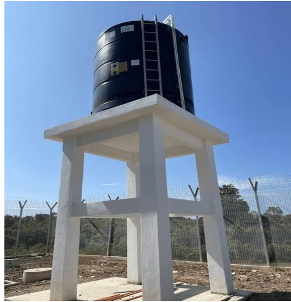
1 no. Mechanised Borehole constructed.
