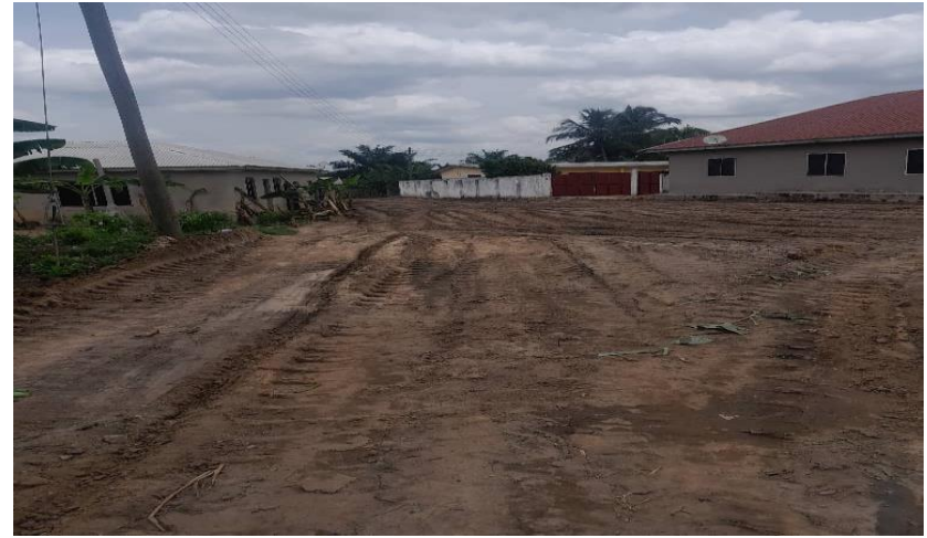
Assin Nsuta township roads reshaped and rehabilitated.
